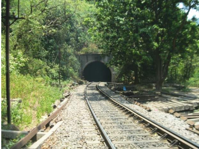
View of Tunnel No. 12 in weathered Granite formation
