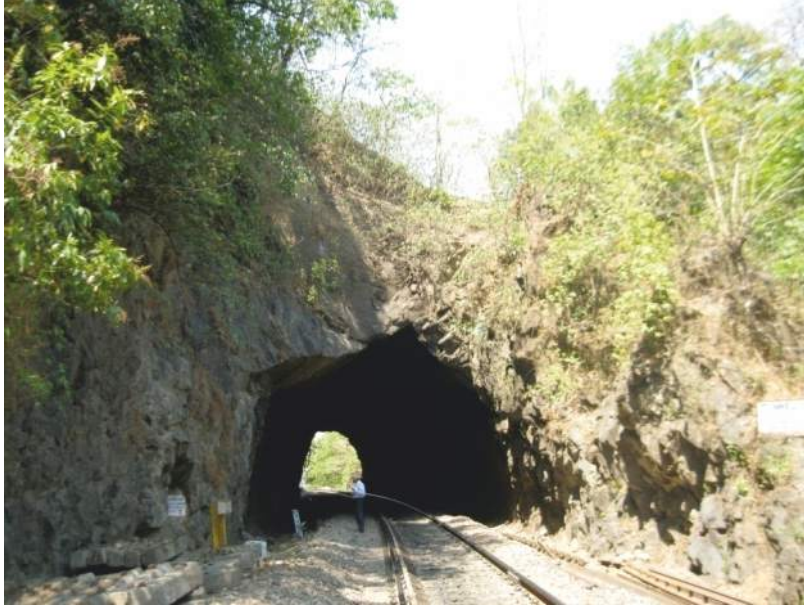
View of Tunnel No.7 in Granite formation
