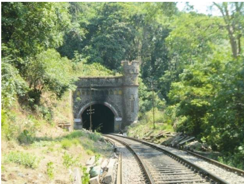
View near Tunnel No. 2
