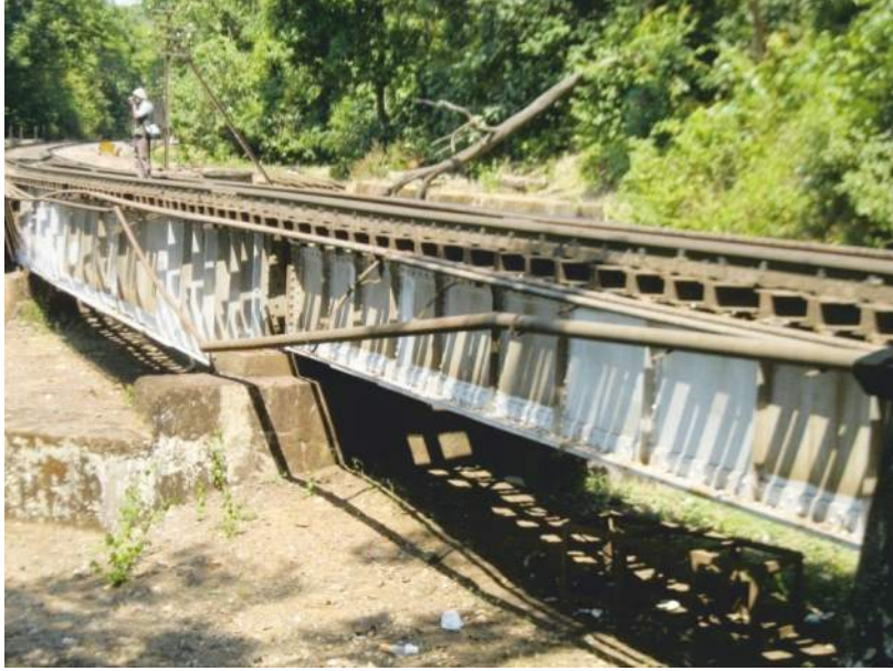
Short Span Girder Bridge in front of Tunnel No 1
