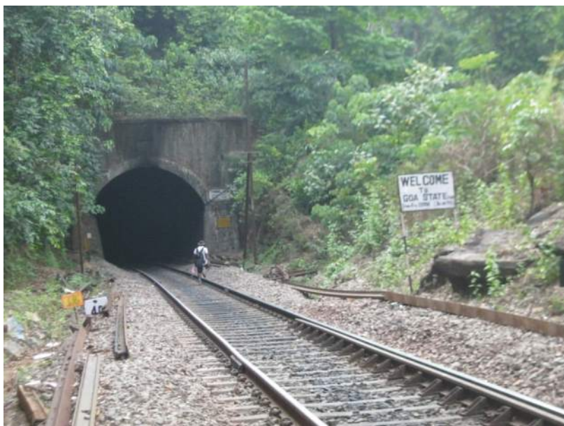
A view of Tunnel No. 4 (Karnataka - Goa Border)
