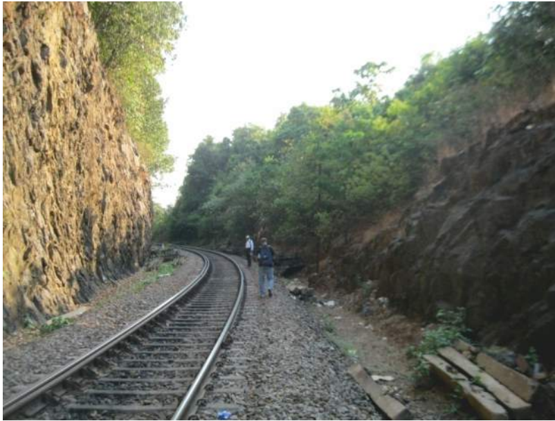
A View of the cutting in Grawec and Metagrawec with chlorite schist's formation after the Tunnel
