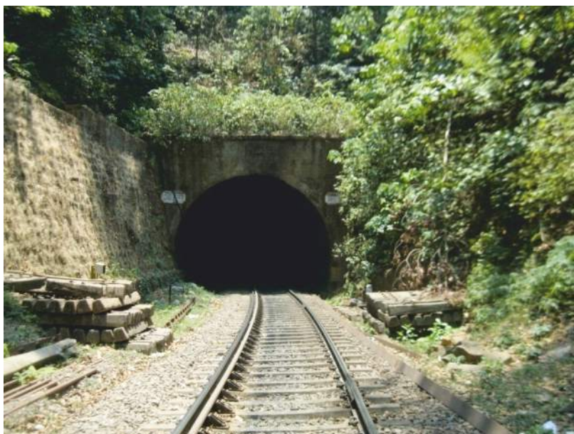
View of Tunnel No. 14 in Grawec formation
