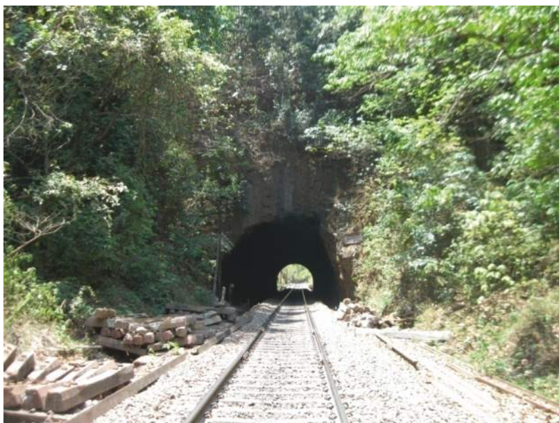
View of Tunnel No. 9 in Grawec/Gabbro formation
