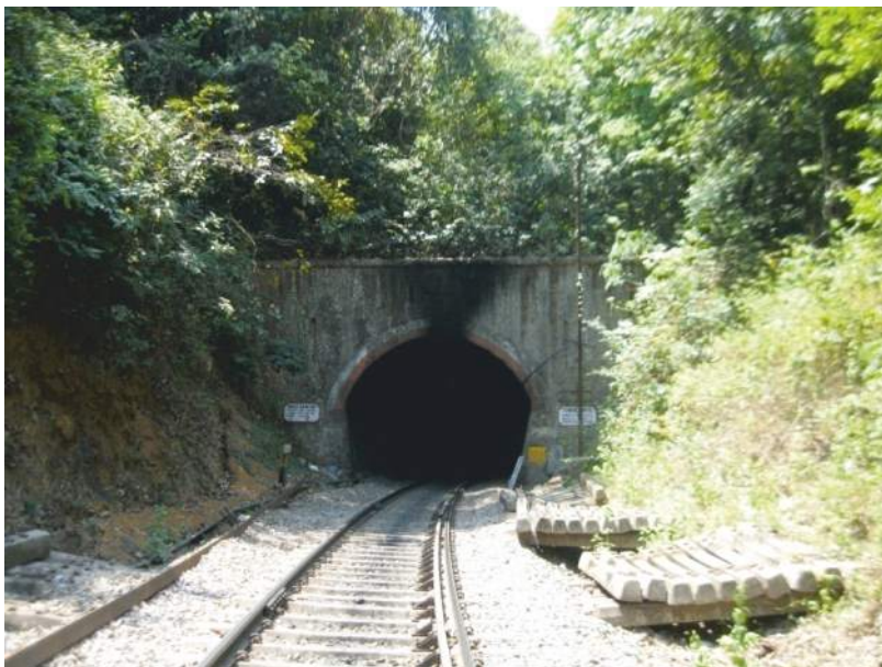
View of Tunnel No. 8 in weathered Grawec formation
