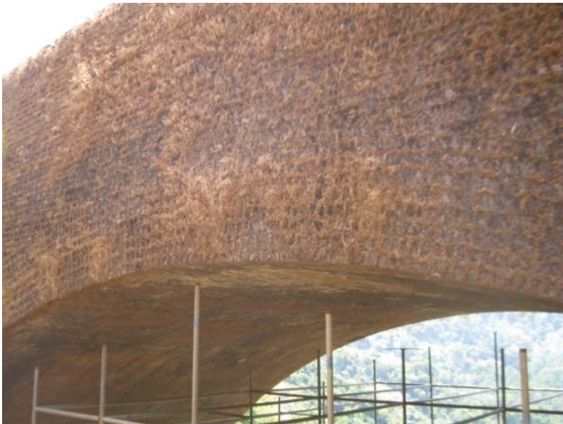
View of existing Arch bridge at the Dudhsagar falls
