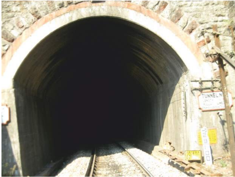
A view of tunnel No. 3
