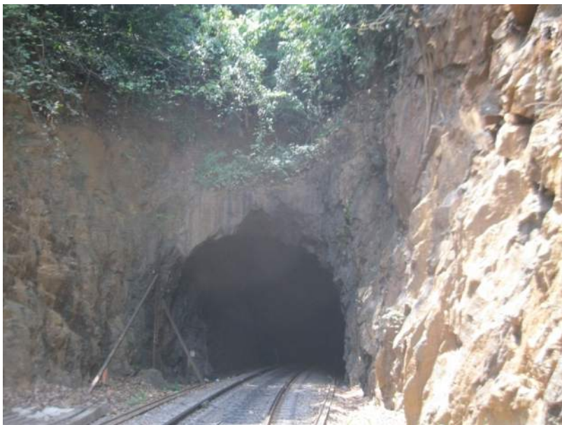
View of Tunnel No. 16 in Grawec and Phylites formation
