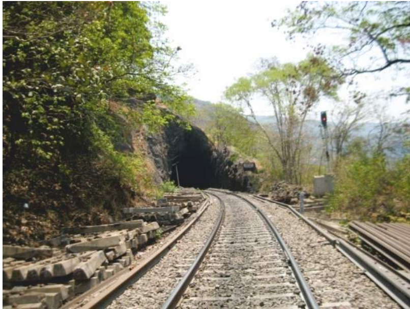
View of Tunnel No. 10 in Granite formation
