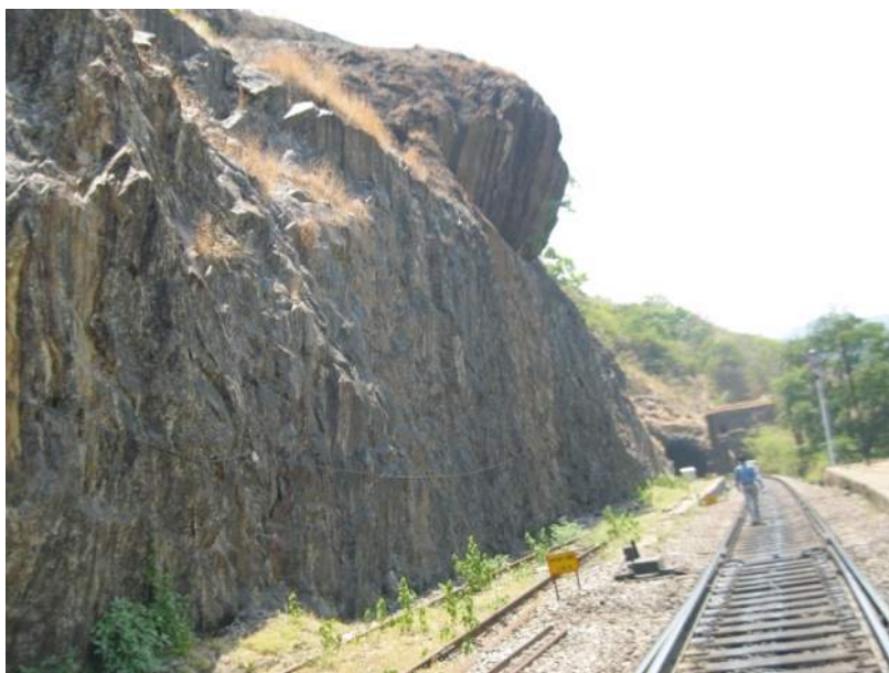
View both cutting and Tunnel No. 10 in Granite formation
