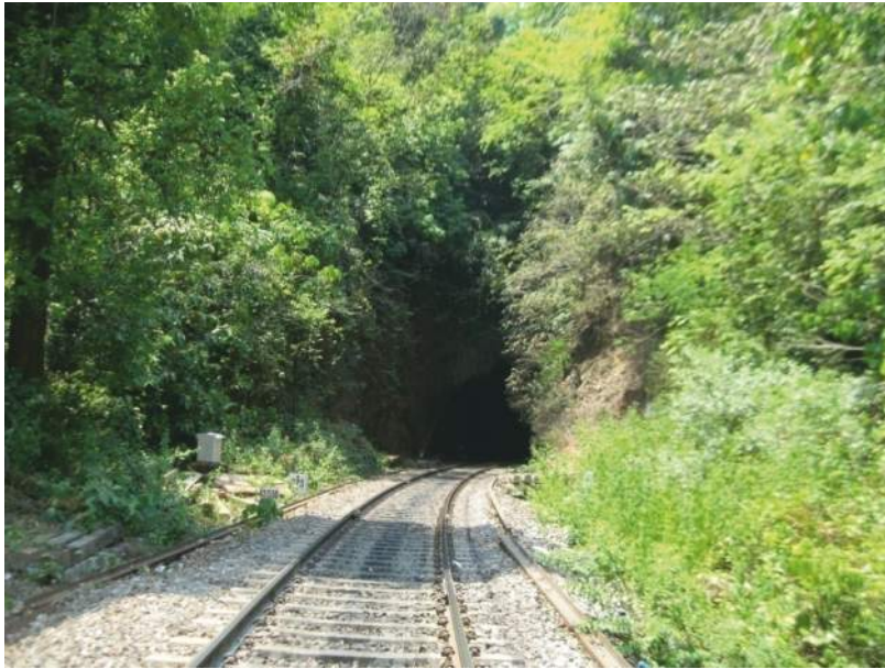
View of Tunnel No. 16 in Grawec formation
