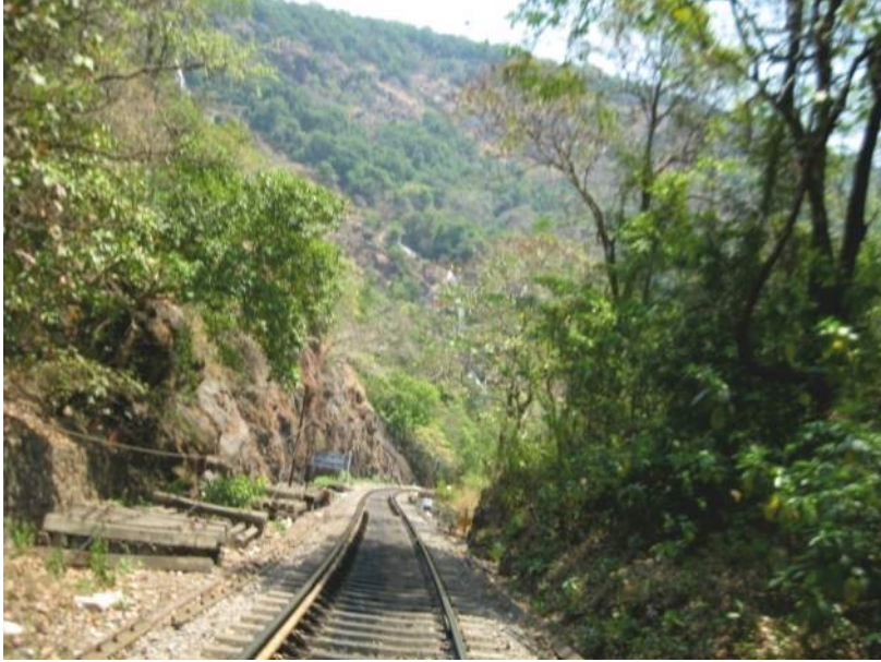
View after Tunnel No. 10
