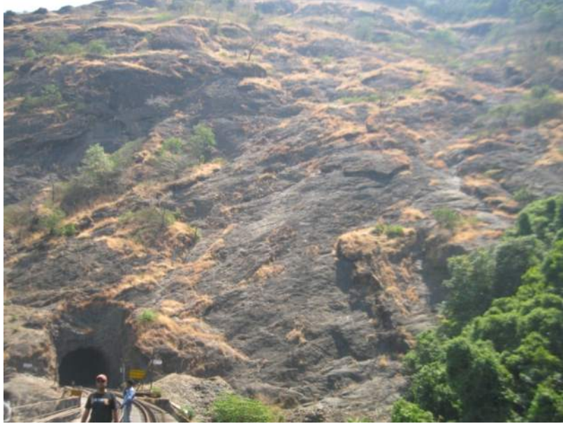
View of Tunnel No.6 in Granite formation
