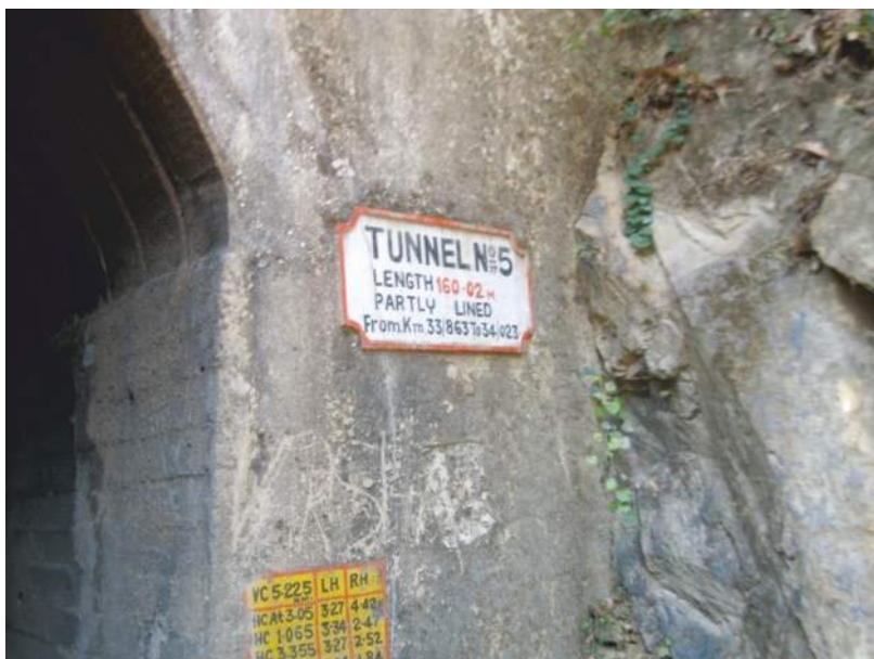
Tunnel no. 5 in weathered Diorite formation
