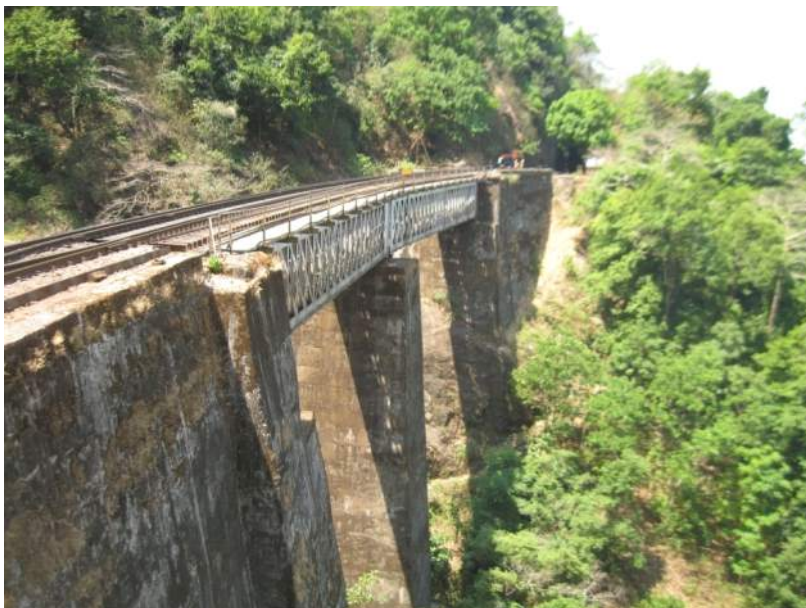
Scalpmnt Viaduct in between Tunnel No 6 and 7
