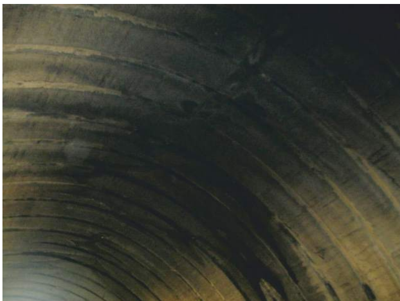
View of the Tunnel lining
