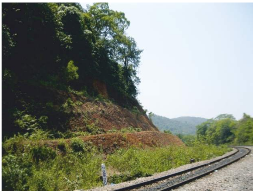
View of stability in red clayey SAND (stepped type)
